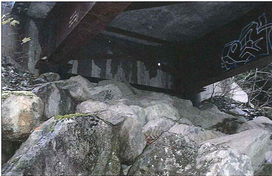
CK2154 Abutment Righth Bank
