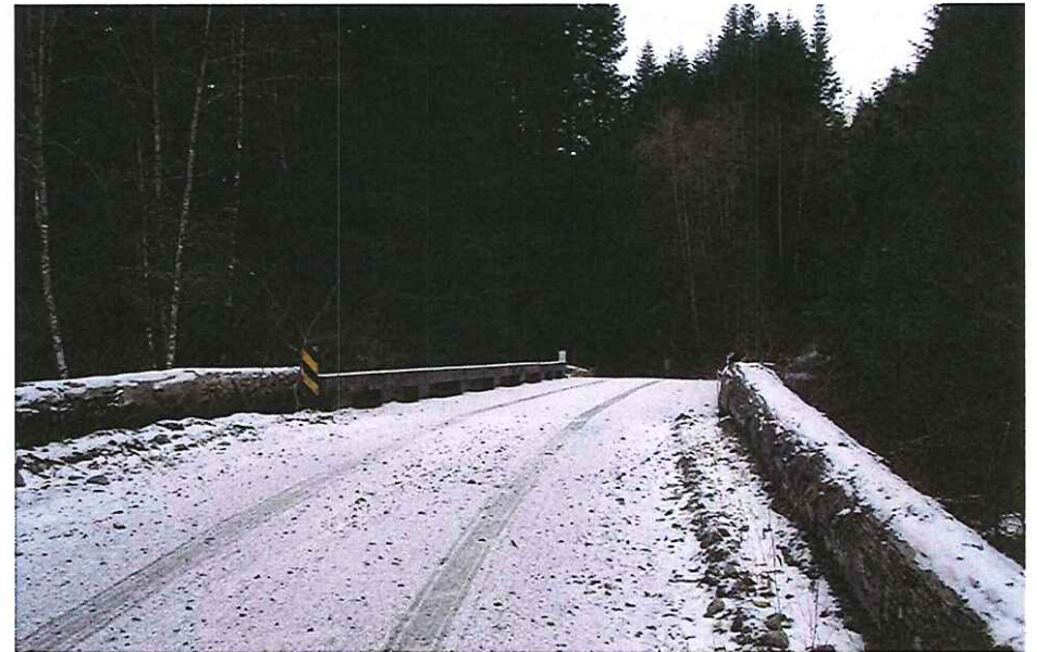
CK2154 Approach Right Bank
