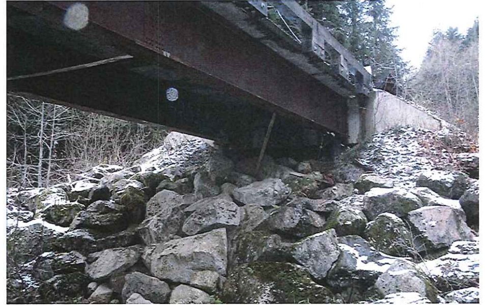
CK2154 Abutment Left Bank
