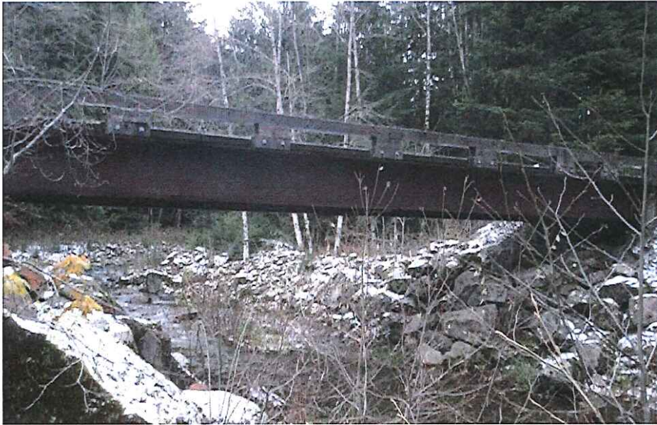
CK2154 Crossing upstream
